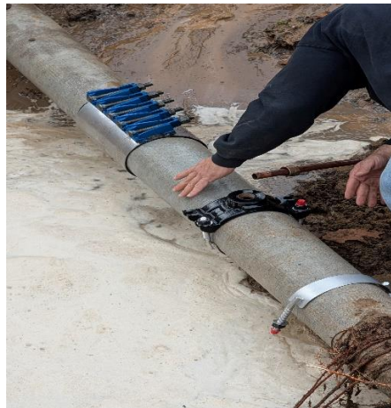
Repair band on a 6" water main at Colorado Road
